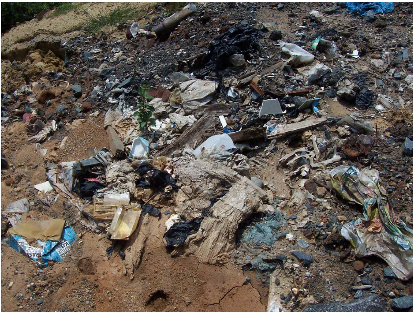
Above, August 29, 2007, Scarborough Landfill south side. Uncovered trash, erosion and spots of leachate.
