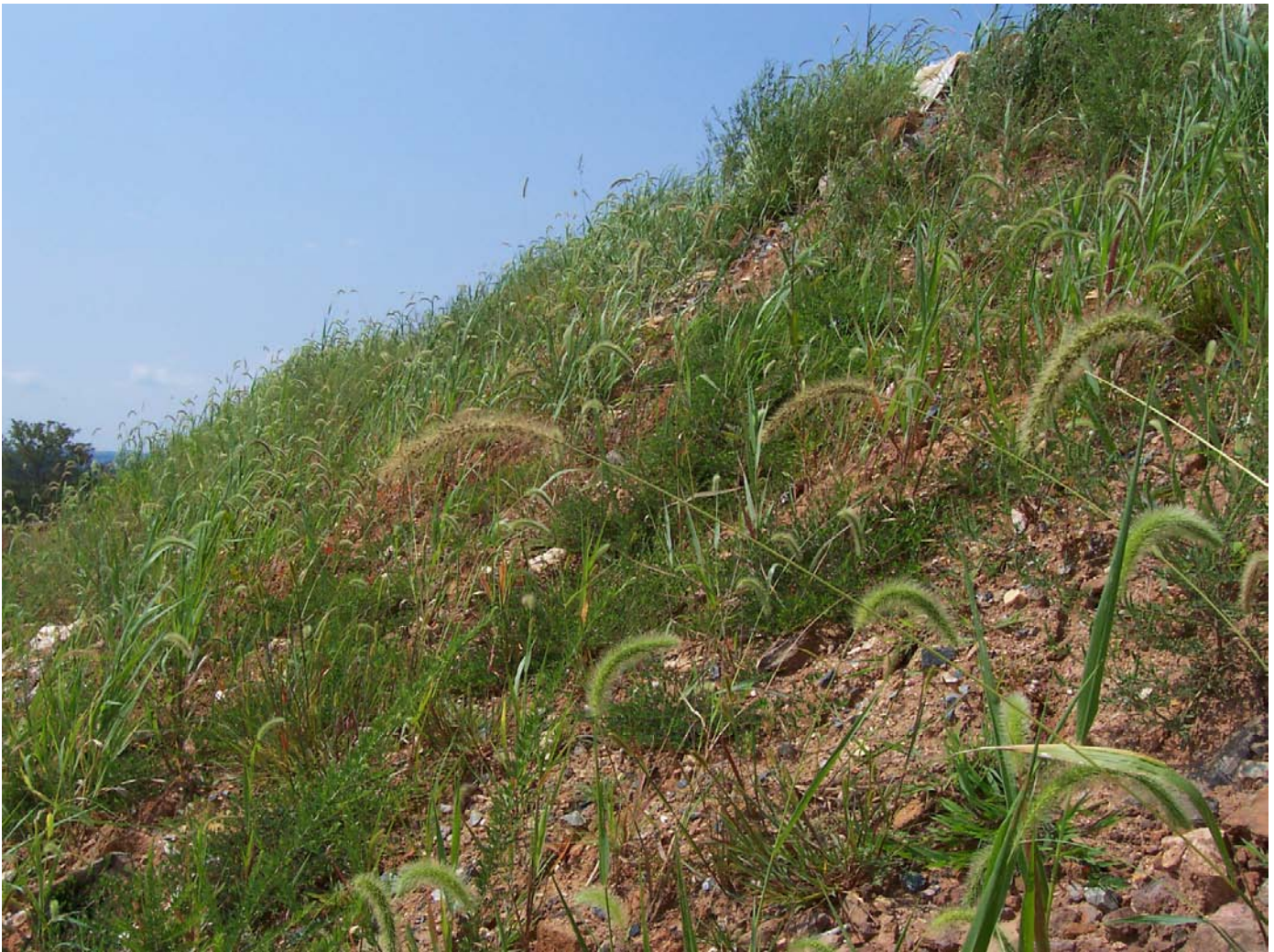
Above, August 29, 2007. Scarboro Landfill south side. Shows steepness of slope. Slope is suppose to be 3:1 this looks approximately 1.5:1 – plus uncovered trash and blown litter.
