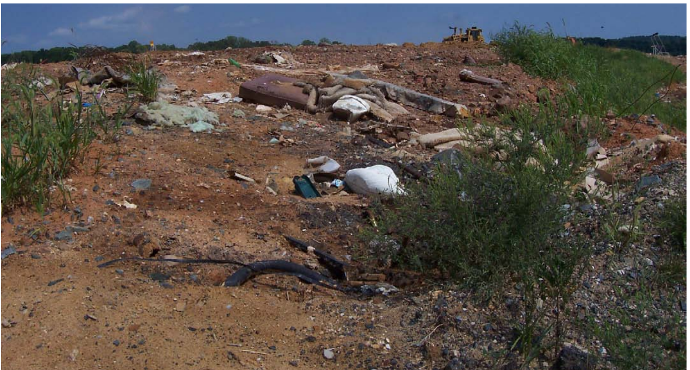
August 29, 2007, Scarboro Landfill south side. Trash never covered – can see workmen at top of ridge – they are working on what can be seen from face – trash just dumped on this side to get out of view.
