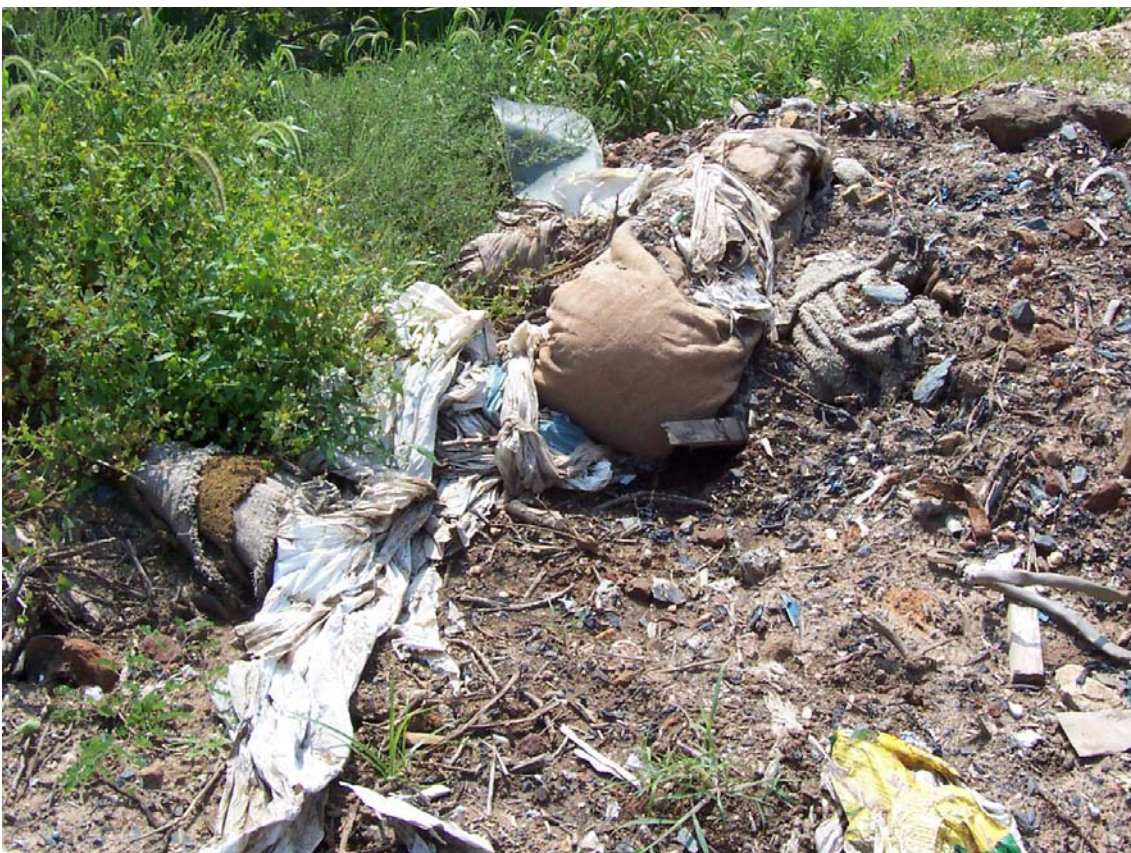
Above, August 29, 2007. Scarboro Landfill south side. Shows steepness of slope. Slope is suppose to be 3:1 this looks approximately 1.5:1 – plus uncovered trash and blown litter.
