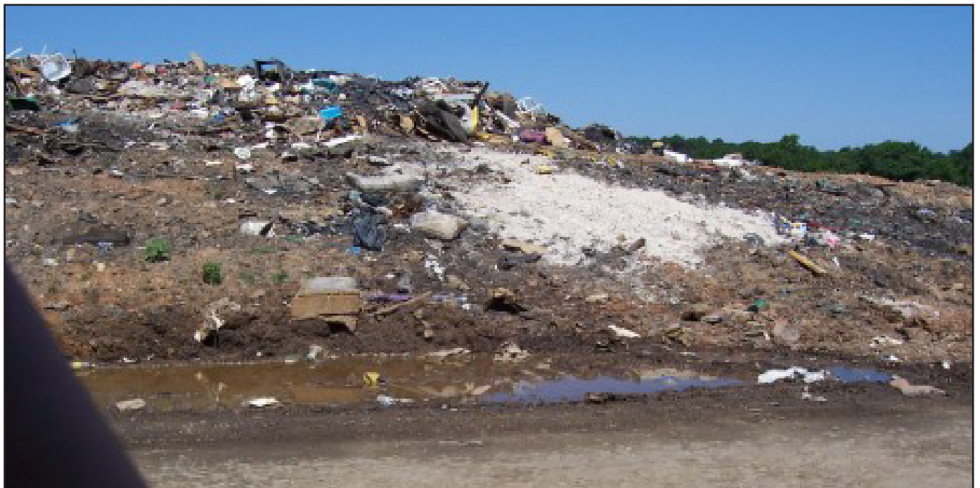
Leachate coming off uncovered trash forming a toxic puddle. Runoff takes it into Deer Creek. Weeds in trash. Weeds are 2 months old. Trash is supposed to be covered daily.
