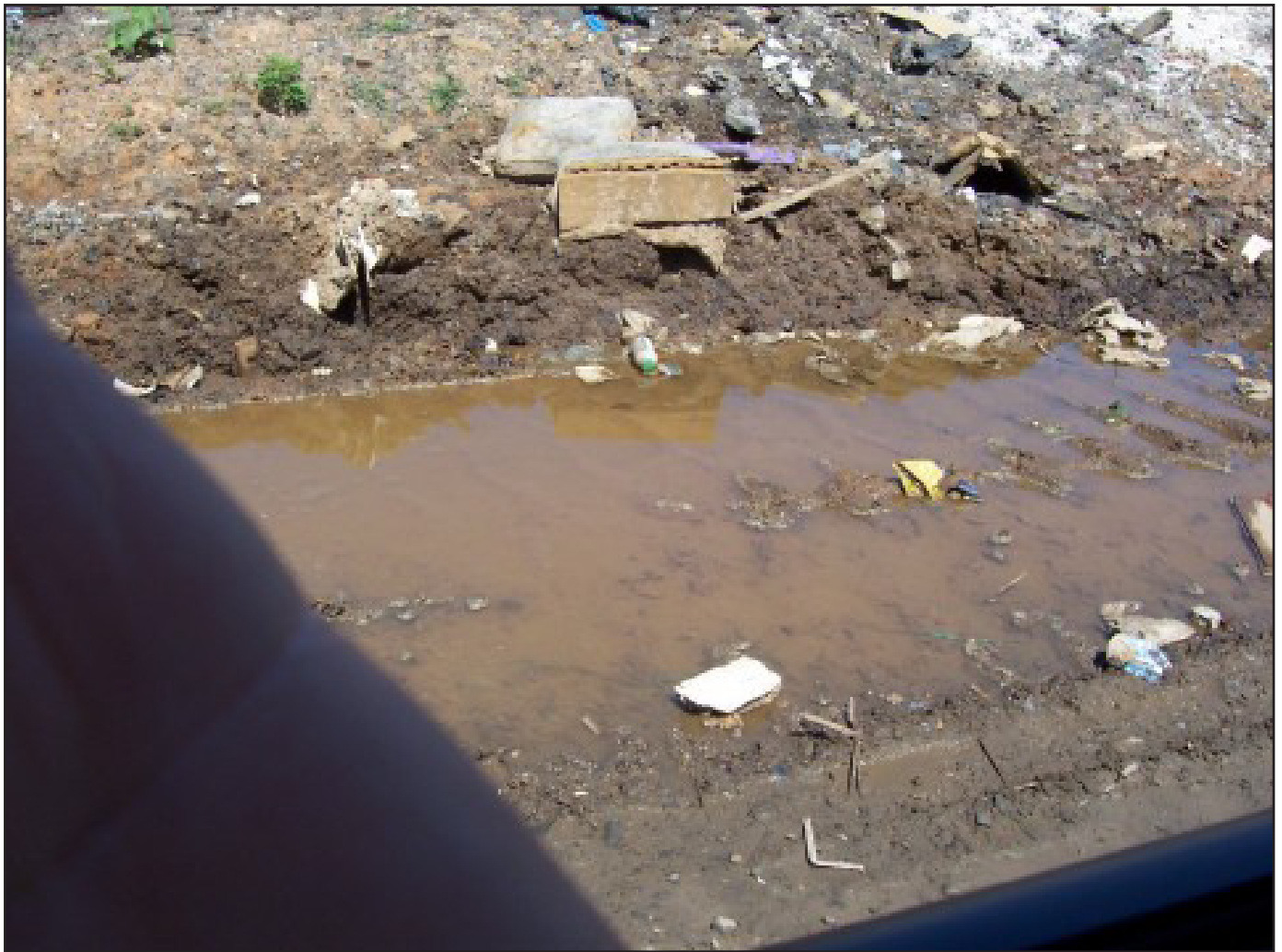
Leachate coming off uncovered trash forming a toxic puddle. Runoff takes it into Deer Creek. Weeds in trash. Weeds are 2 months old. Trash is supposed to be covered daily.
