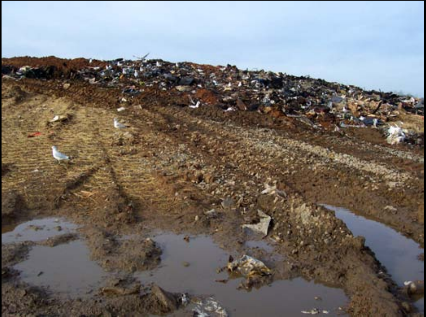
Landfill & Southside Jan 10 2008 006. Ponding water, inadequate daily cover
