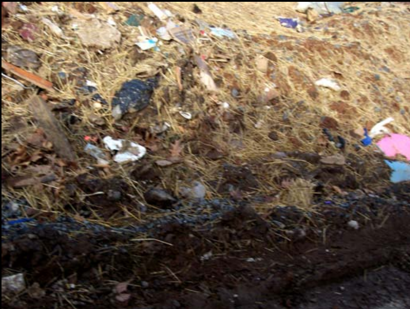
Landfill & Southside Jan 10 2008 010. Seeded over exposed garbage - inadequate intermediate cover (should be 1 foot)
