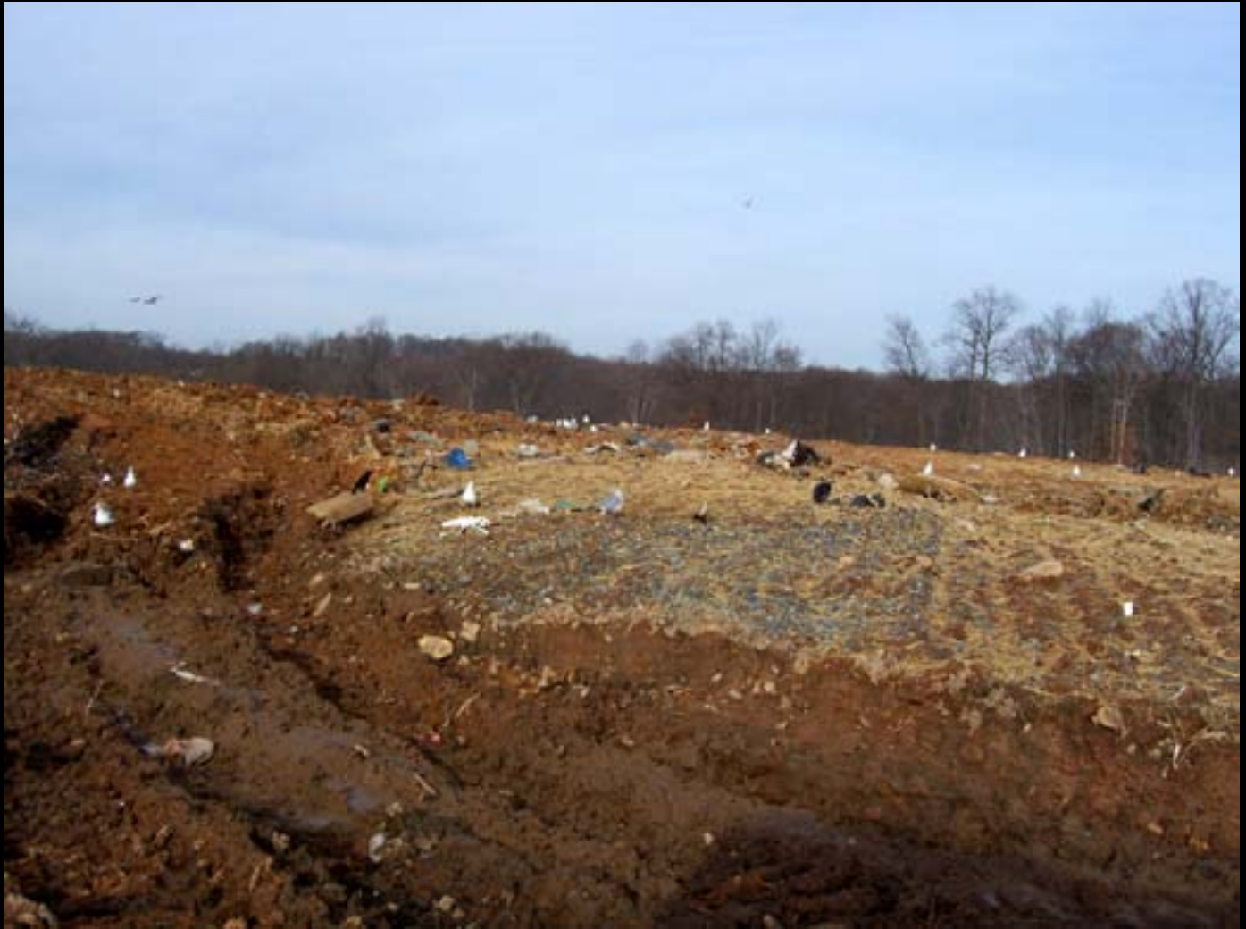
Landfill & Southside Jan 10 2008 009. Straw over seeded area no intermediate cover (1 foot)
