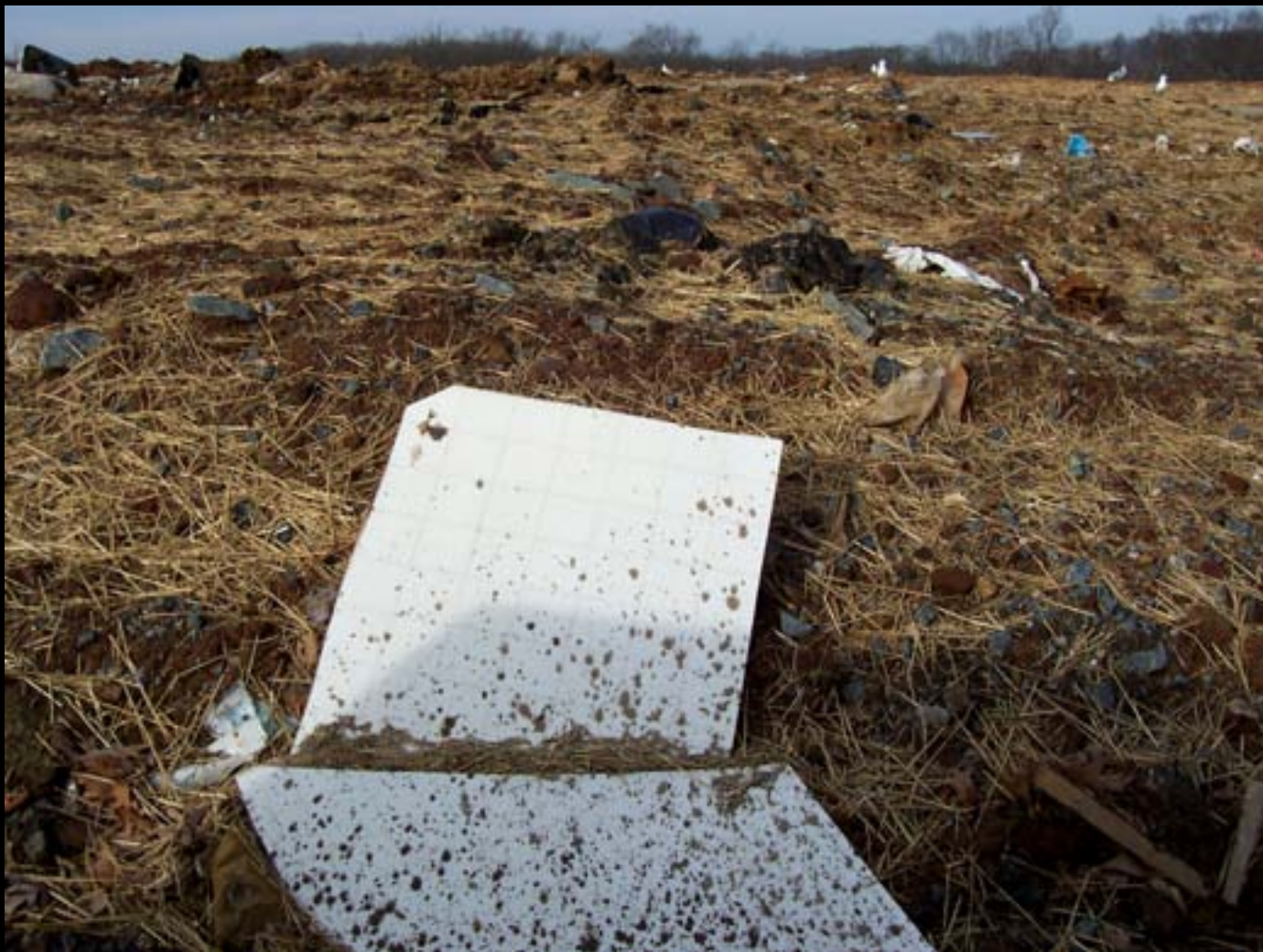
Landfill & Southside Jan 10 2008 013. Seeded over exposed garbage - inadequate cover - attracts vectors.
