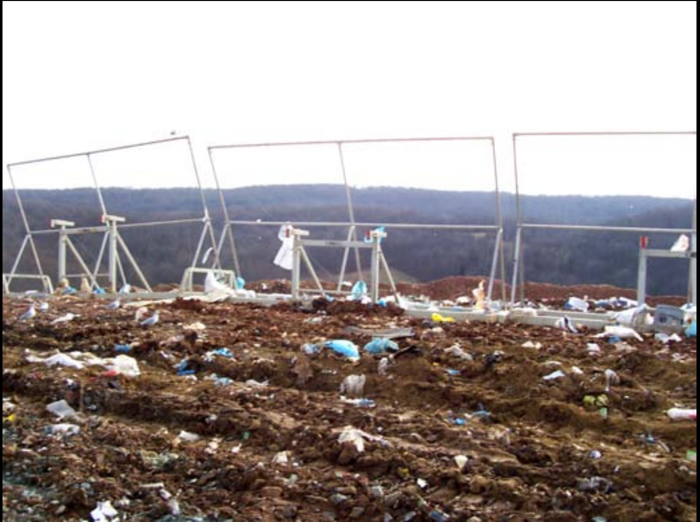
Landfill & Southside Jan 10 2008 004-1. Inactive working face - no 6' of cover.
