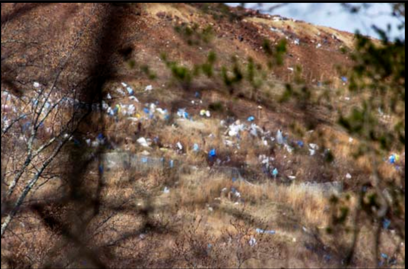
Southside. Steepness of slope. Areas without vegetation allow erosion causing gullies and instability. Uncovered, windblown trash. This is a completed cell, supposed to be finished, as good as it gets.
