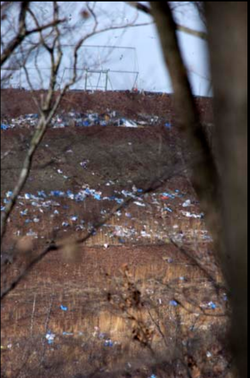
Southside supposedly finished area with exposed trash, wind-blown trash, blue recycle bags (do the people who bother to use them know this is where they wind up?) unstable banks, deep erosion.
