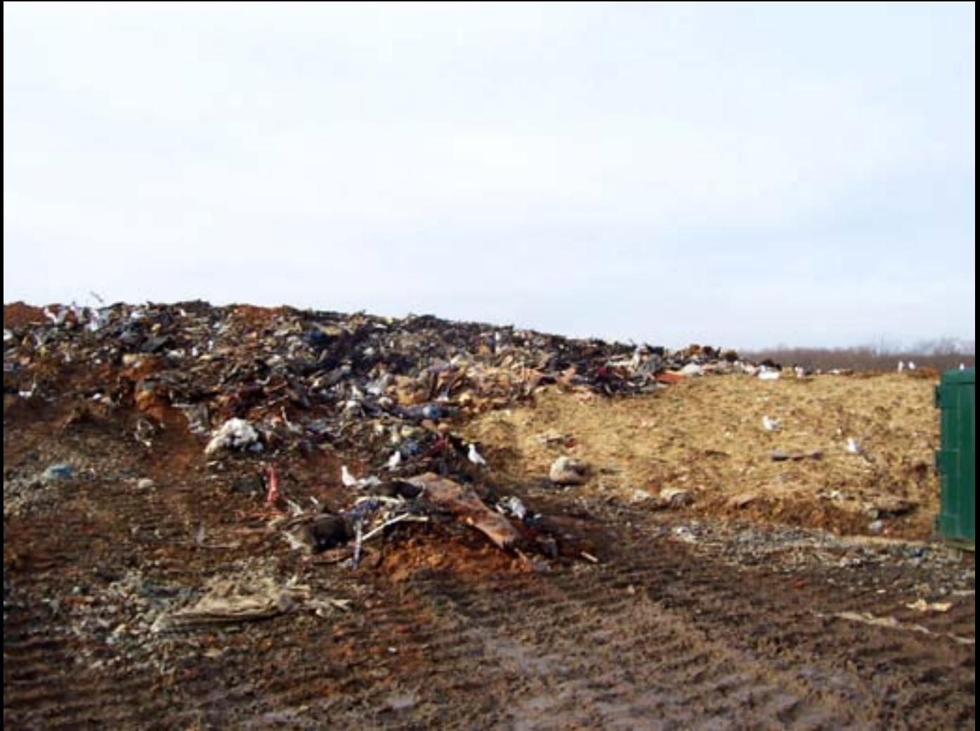
Landfill & Southside Jan 10 2008 008 Inadequate daily cover. Straw area already seeded over uncovered trash.
