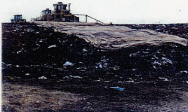
Installing the Tarp-O-Matic ADC
