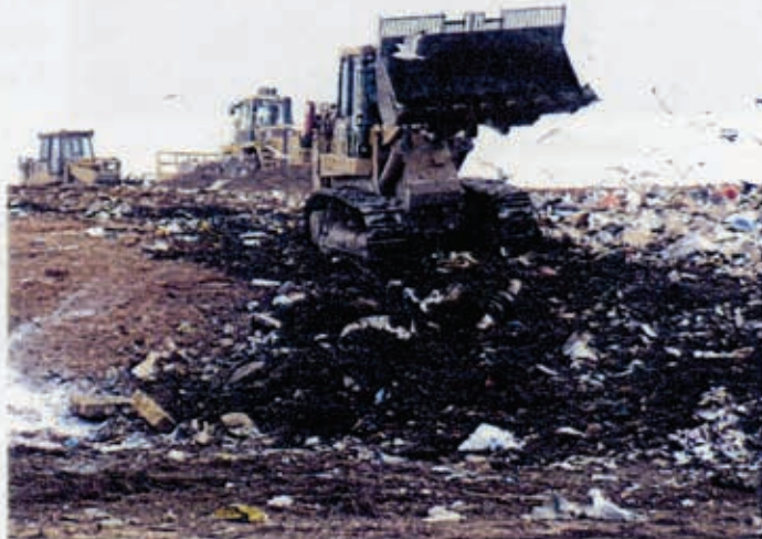
Spreading Intermediate Cover at Workface
